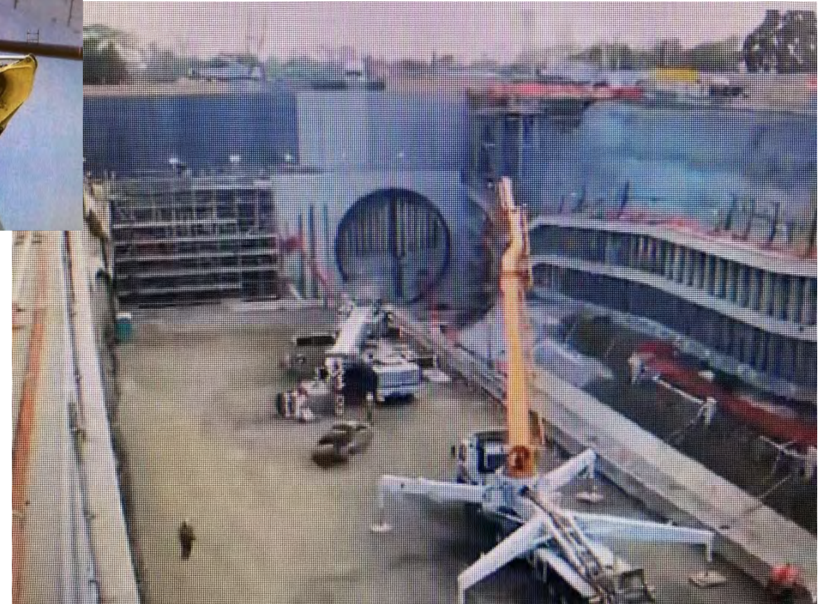
Cofferdam for TBM Entry Point
