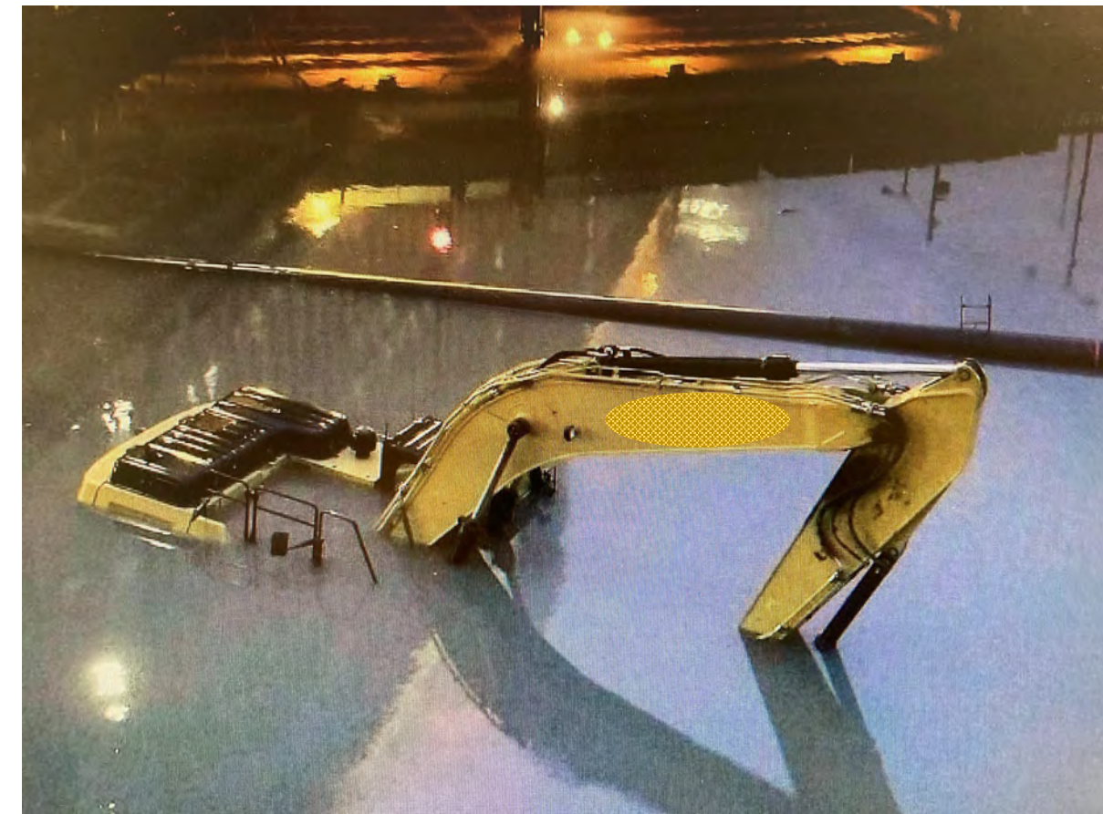
Coffer dam over topped by storm
