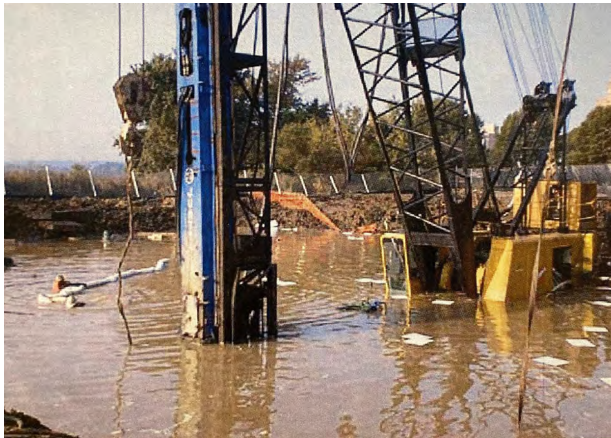
Coffer dam failure
