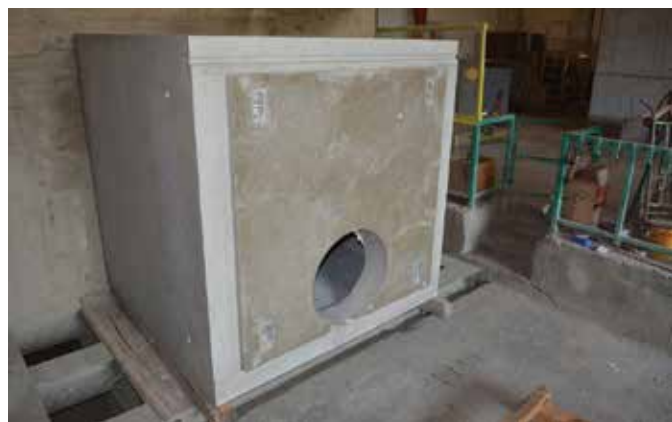
Fig. 1: The bottom of an upper-tier module. The relief (darker raised area) will nest inside the walls of the module below. The circular opening will allow workers to access the module below and bolt the two together through holes formed using PVC pipe near the four corners of the face. The reveal near the top of the photo will be fitted with an expansive waterstop immediately before the module is installed in the dam
