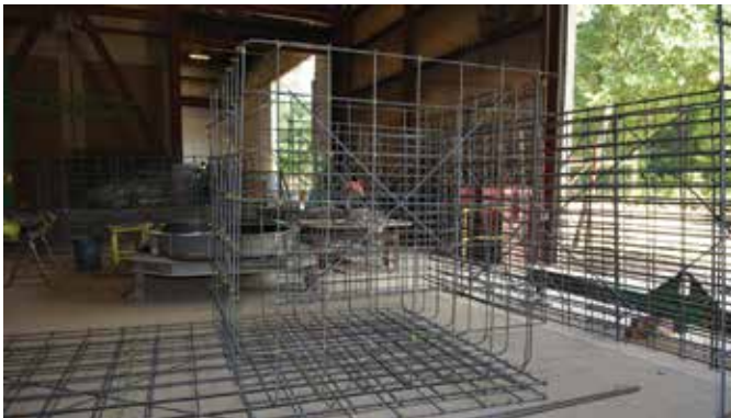
Fig. 2: A reinforcement cage for an upper-tier module
